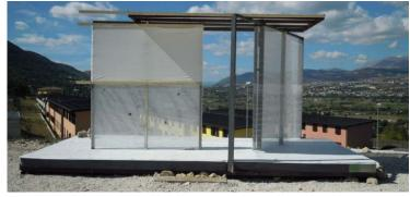
The pavilion was made from "recycled" old steel frames that were found on site. For the partioning walls and floors high-tech textiles made from artificial fibre were used. – With its design and light appearance the pavilion was to evoke the appearance of a Japanese teahouse.
