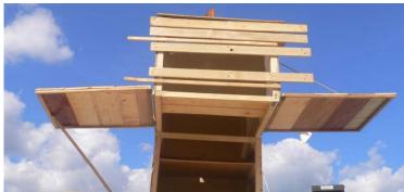
The Micro-Library was made form leftover timber and wood. As a main material, old "bancali" – the standard transportation palets – were used and recycled. – The Micro-Library itself was conceived to be mobile and transportable. Such it is able to change its position according to local needs, season, and frequence of use.
